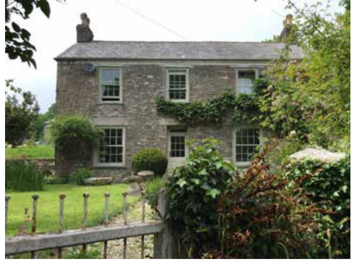
Double-fronted. Granite dressings. Front garden within stone boundary wall.
