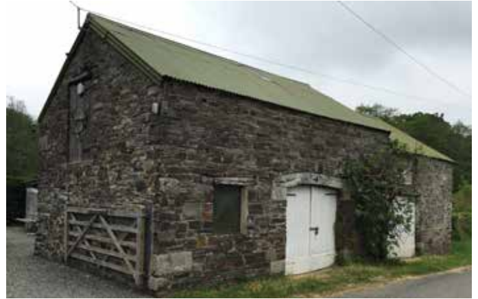
Barn ensemble with random rubble walls and modern corrugated sheet roof.
