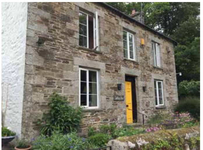
Above: Random rubble wall without dressings to window opening. Slate roof.
