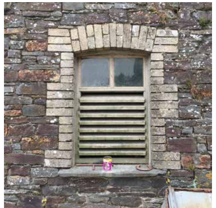
Buff brickwork used in place of granite for window dressings.
