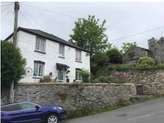
Limewashed walls with the stone texture showing through.
