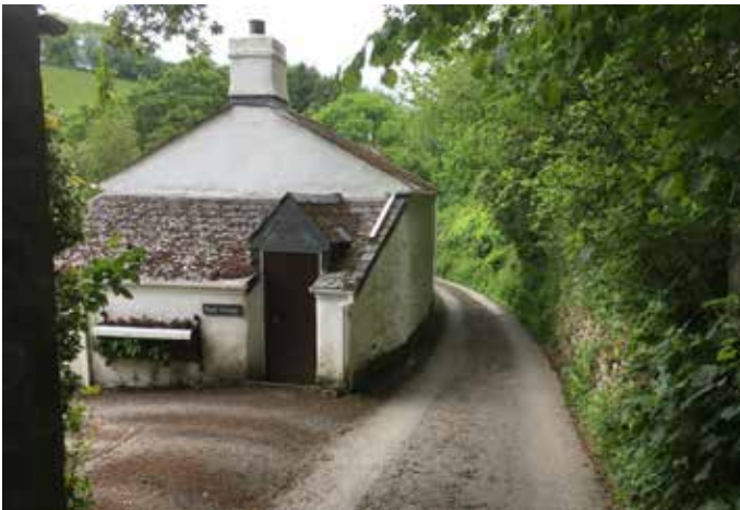
Narrow lane. Shallow, one room deep plan. Improvised entrance. Limewash on rubble walls.
