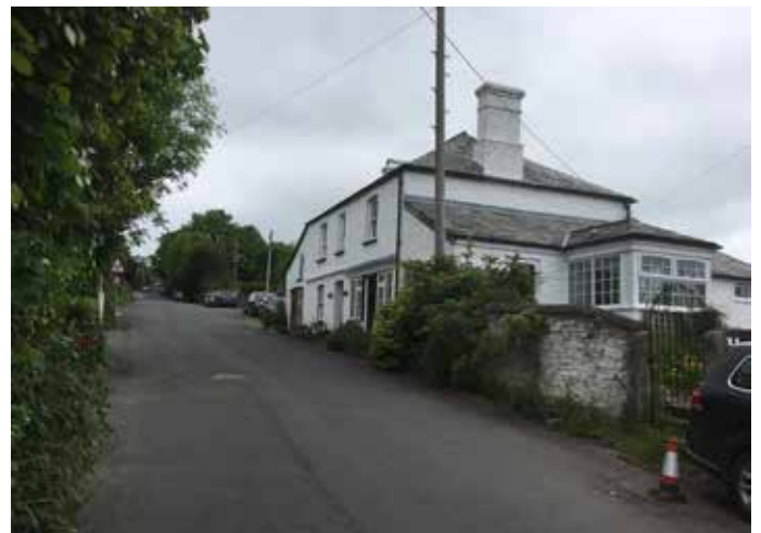
Larger building climbing the hill. Limewash, hipped slate roofs.
