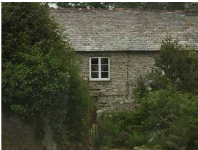
Above: Random rubble wall without dressings to window opening. Slate roof.
