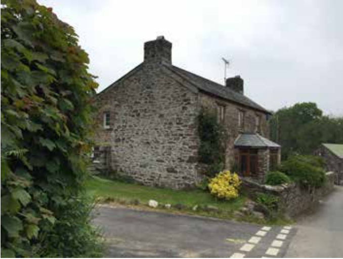
Low pitched slate duo-pitch roof. Symmetrical front. Asymmetrical gable. Random rubble.
