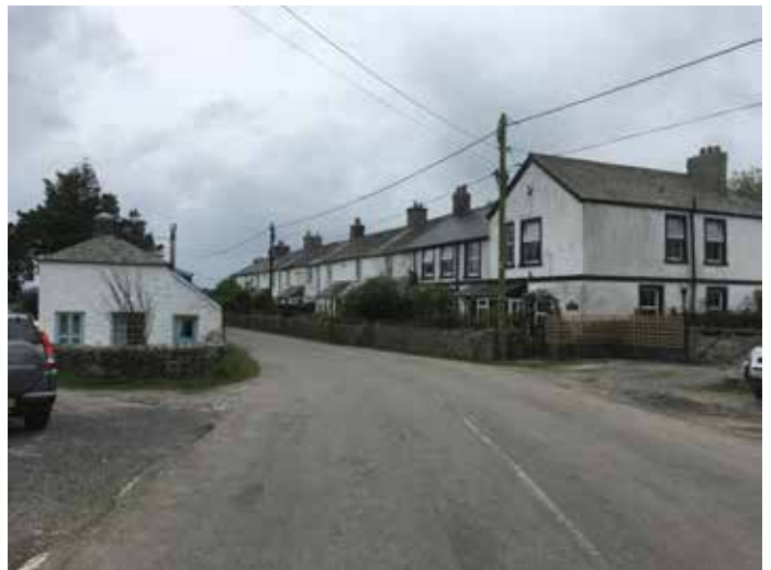
Terraced workers' housing on top of the Moor. Linear terrace with terminating gabled house.
