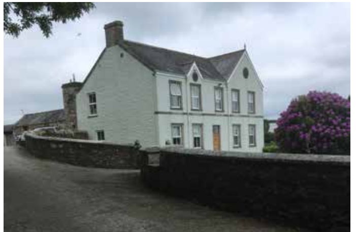
Modified & extended double-fronted house embellished with gables.
