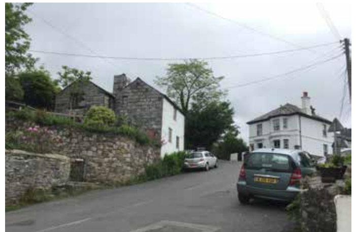
Random stone retaining wall, slate hanging & limewash.
