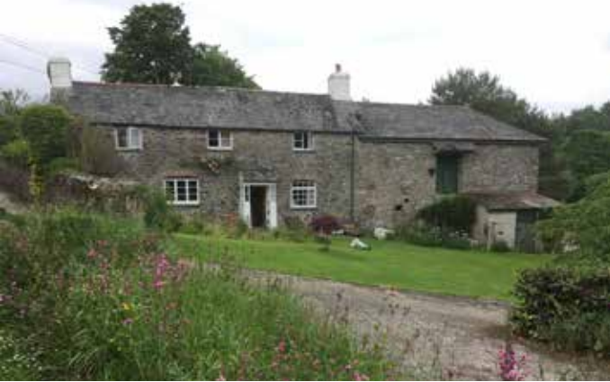
Farmhouse with longitudinal barn with low pitched hipped roof.
