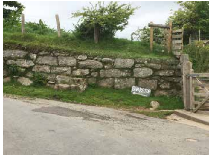
A hedge built of large field and quarry stones.
