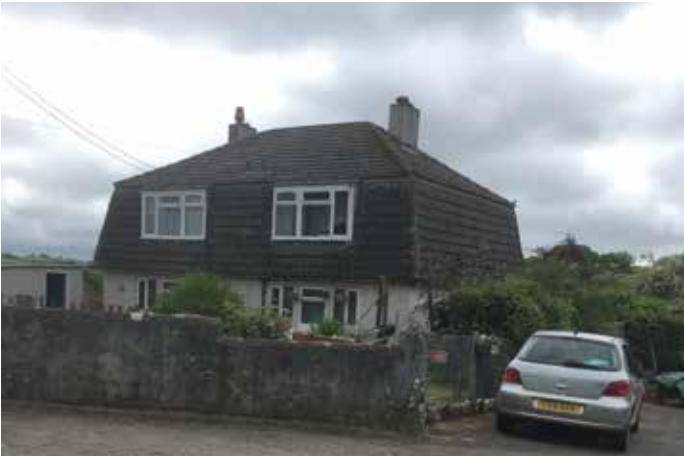
A pre-fabricated 'Cornish Unit' creates an isolated suburban effect.
