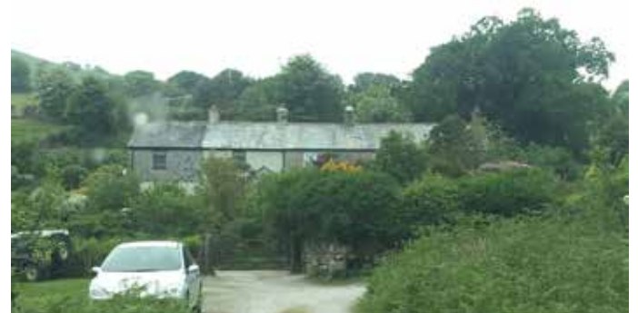
Slate hung terrace sheltered by trees on the edge of the Moor.
