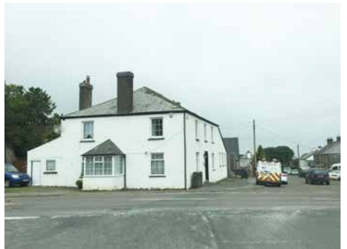
Shop and house on a major crossroads.
