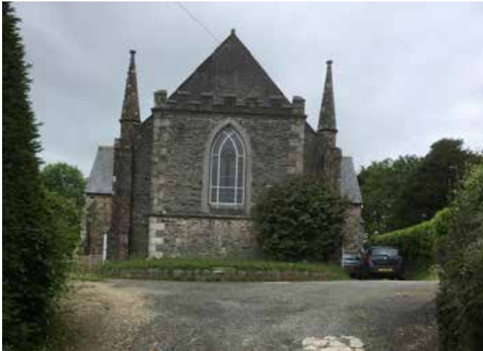
Church viewed from the main road. Occupies the rising ground and presents a symmetrical face.
