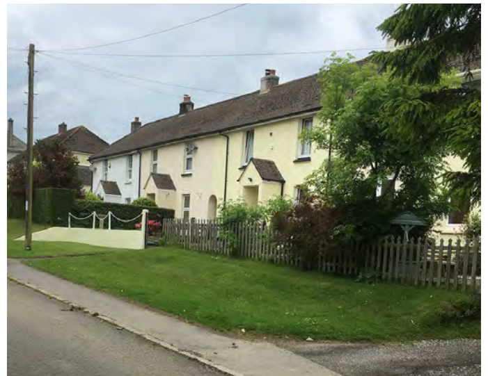
Workers' terrace. Simple double-fronted cottages. Low, continuous eaves. Shared 'areas' leading to back gardens
