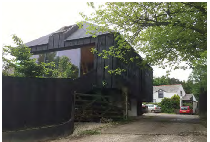
A modern house near Upton Cross uses timber cladding and non-domestic form to differentiate it from the traditional farmhouse beyond. This arrangement is analogous to the traditional house and barn in a farmyard setting.
