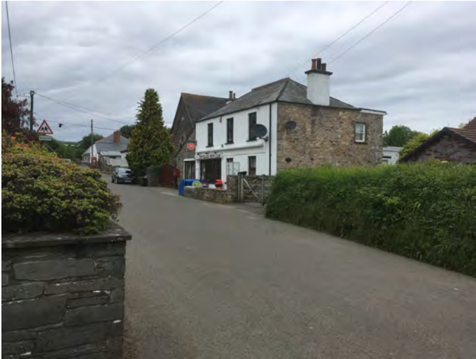
Former Post Office with the low pitched and hipped roof often found on larger, more prestigious buildings.
