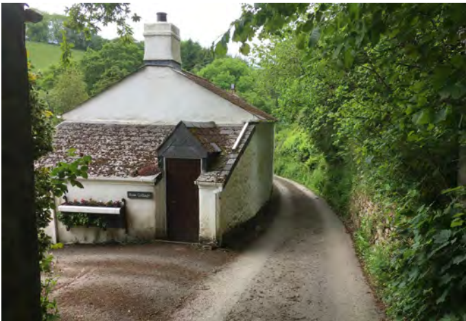
Narrow lane. Shallow, one room deep plan. Improvised entrance. Limewash on rubble walls.
