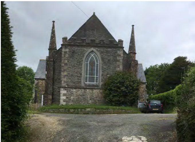
Church viewed from the main road. Occupies the rising ground and presents a symmetrical face.
