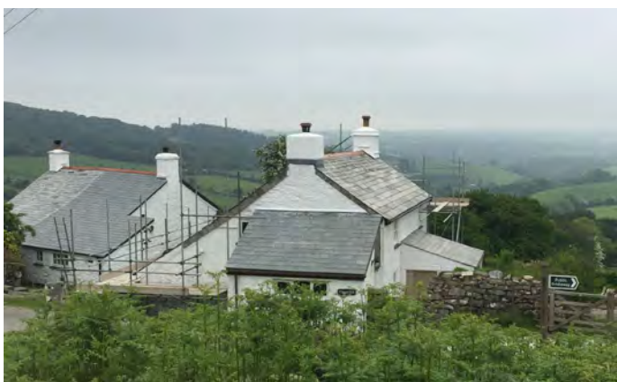
Houses with mono-pitch additions occupy available plots on the slope up to the Moor.
